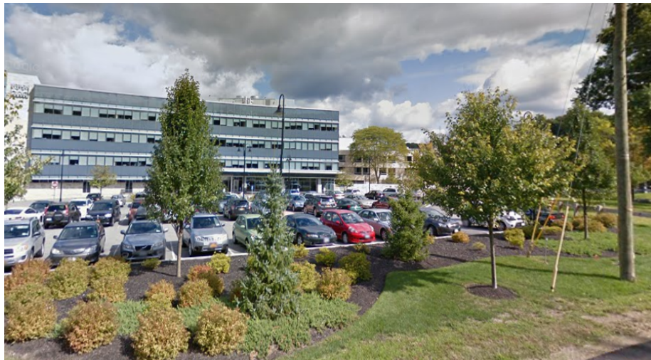
Photo 1: View of NYPH from Route 202/35/Crompond Road looking northeast
