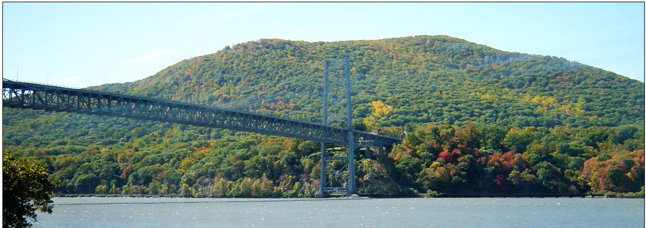
Bear Mountain Bridge (Town of Cortlandt)
