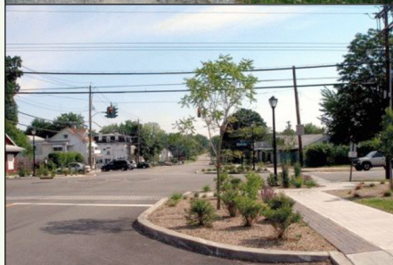
Broadway Streetscape Improvements Before (above) and After (below) (Town of Cortlandt)
