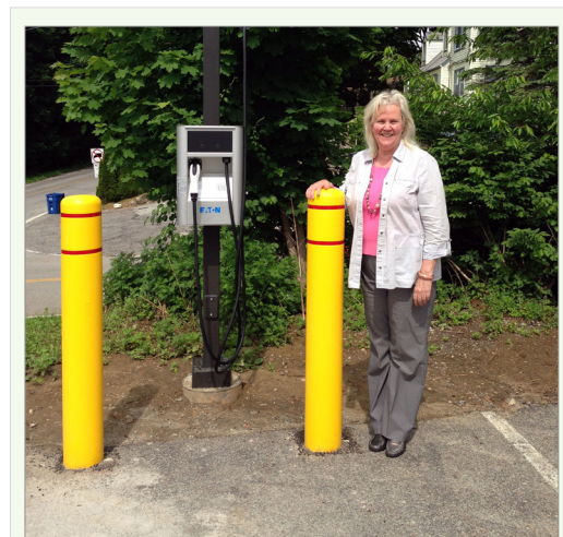
Supervisor Linda D. Puglisi in Front of the EV Charging Stations Installed at Town Hall in 2014 (Dani Glaser)
