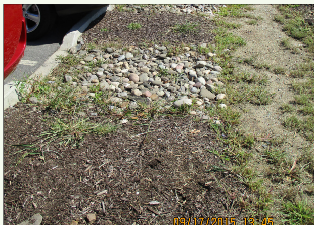
Stormwater Swales along Route 6 (AKRF, Inc.)
