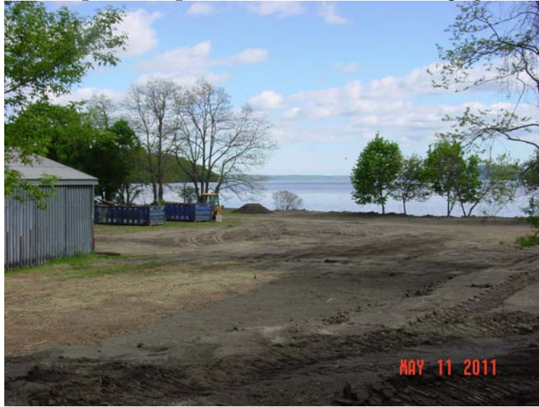
Grading at the Sturgeon Boat Club/Former Martin Property
