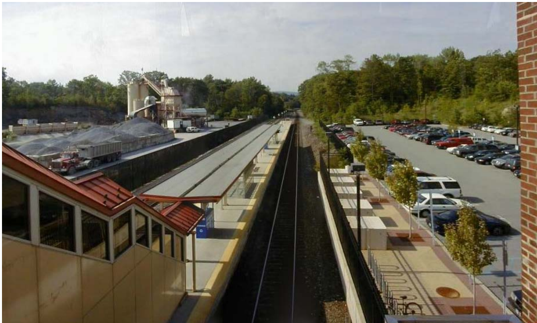
Cortlandt Manor Train Station
