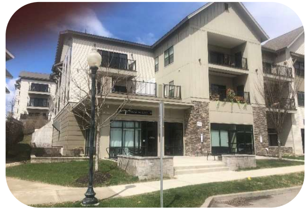
Three story mixed use building.
