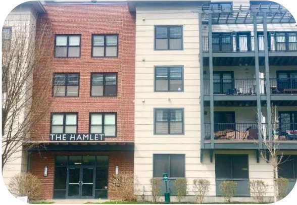
Four story plus penthouse mixed use building.
